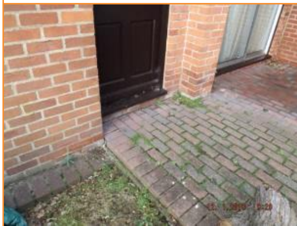
4.1: Major leakage along the side of external door whilst house is pressurised.
