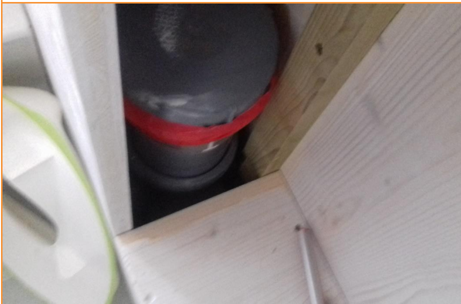
A1.4 Admittance valve in family bathroom temporarily sealed for duration of testing. A second admittance valve in a WC was also sealed
