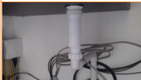
A1.4 Admittance valve in family bathroom temporarily sealed for duration of testing. A second admittance valve in a WC was also sealed
