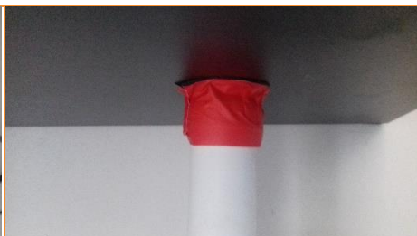
A1.4 Admittance valve in family bathroom temporarily sealed for duration of testing. A second admittance valve in a WC was also sealed
