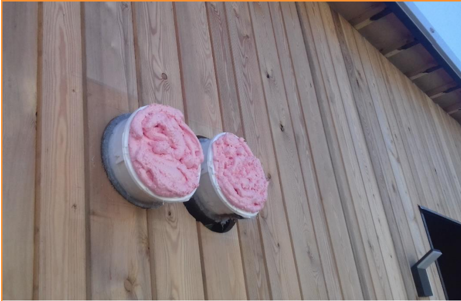
A1.3 MVHR grilles sealed externally
