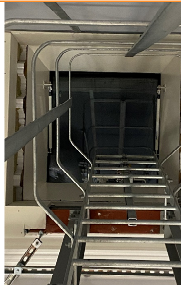
A1.8) Verification that roof access hatch was shut for the duration of acceptance testing
