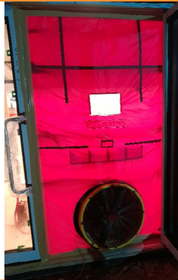
A1.2) External view of test equipment mounted in bag door system in L1 Main Entrance
