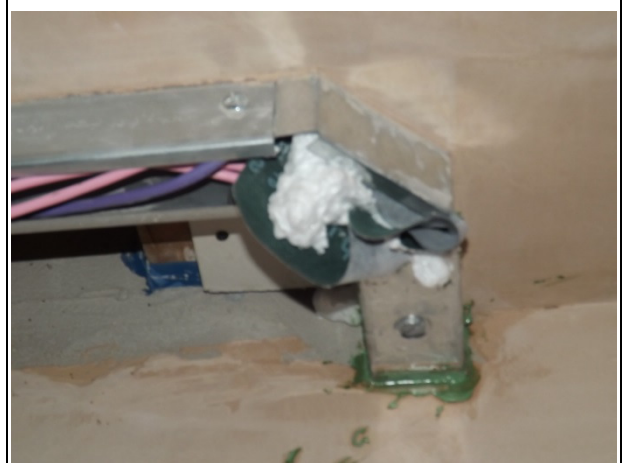
P15) 2" trunking sealed with foam and around with mastic – more than once (item 9)
