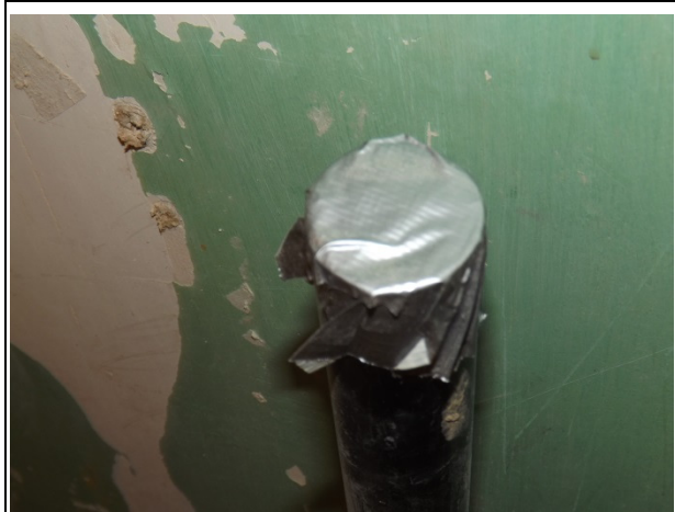
P5) Top of incomplete pipe sealed for test
