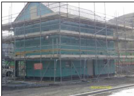
Initial test, April 2010 At completion of timber frame Achieved 0.29 AC/hr @ 50 Pa
