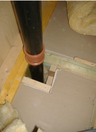
22) Hole around SVP into loft
