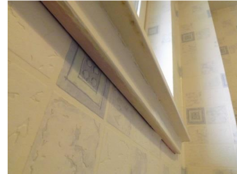
2) Under window sills
