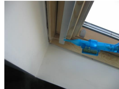
10) Checking rooflight for leaks
