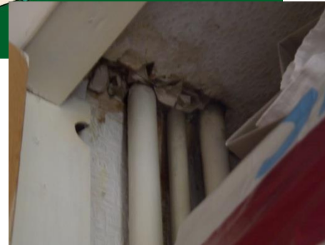
24) Unsealed pipes & cables through top of airing cupboard
